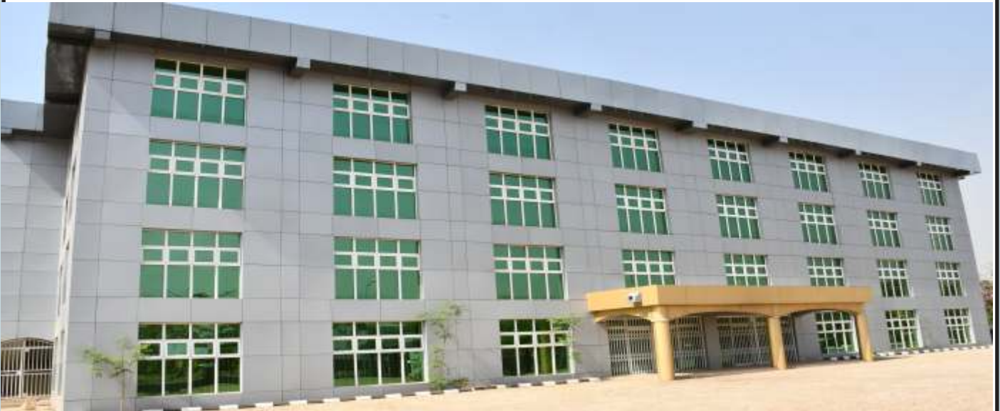
New Office Building of the Court, located at Gudu District – Abuja.
